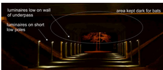
Figure 5.3. Installation of luminaires on short poles for mitigating the effect of ALAN on a commuting route through an underpass in the Netherlands (the same place in daylight and at night). This solution was proven as efficient for P. pipistrellus but not for the low-flying species M. daubentonii (© F. BREKELMANS).
